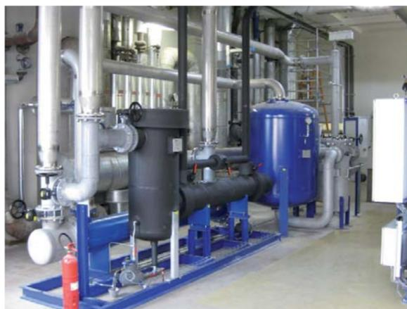
By precooling the compressed air, an EVERDRY adsorption dryer of the 3400 FRA type can even reliably master an overload of up to 5,000 m³/h.
