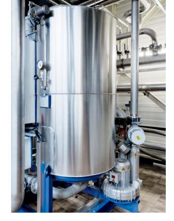
Depending on the requirement, the warm, dry blast air, which accrues during cooling of the heated desiccant, can be used for room-heating or discharged to the atmosphere.
