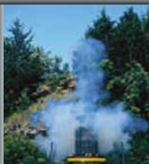
Flameless Venting with FlamQuench II™
