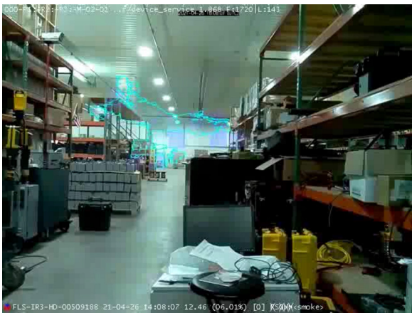
Smoke detection at 200 feet.
